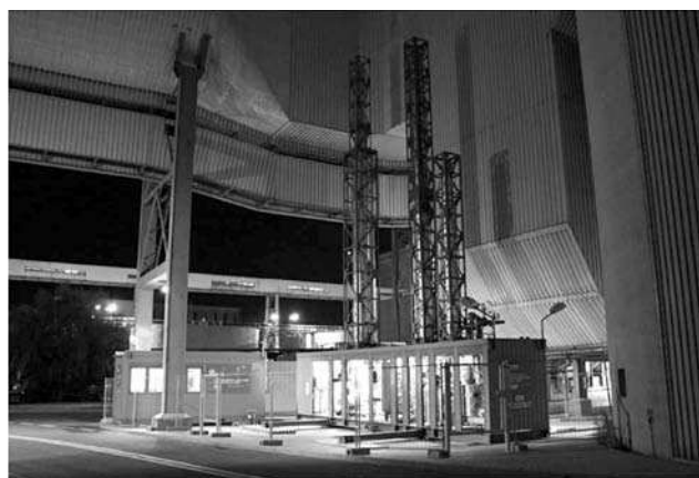
Fig. 2. Pilot plant during night research campaign in Laziska Power Plant
