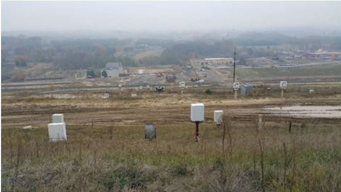
Fig. 2. Surface of the earth embankment around the Želazny Most reservoir
