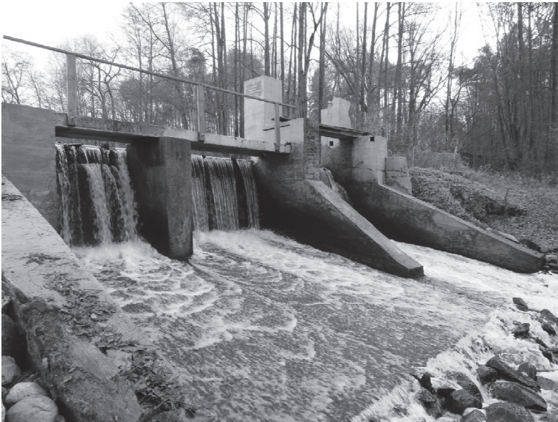
Fig. 2. View on the weir in Dobrzyca on the Głomia river
