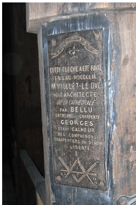
Fig. 4 A plaque commemorating Viollet le Duc and the builders of the spire, mounted in the attic on the central wooden pillar of the spire structure, photo D. Mączyński 2009
