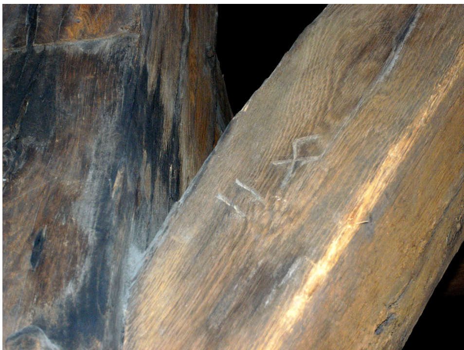
Fig. 3 Carpentry marking on an element of the roof truss of the Notre Dame cathedral, photo D. Mączyński 2009
