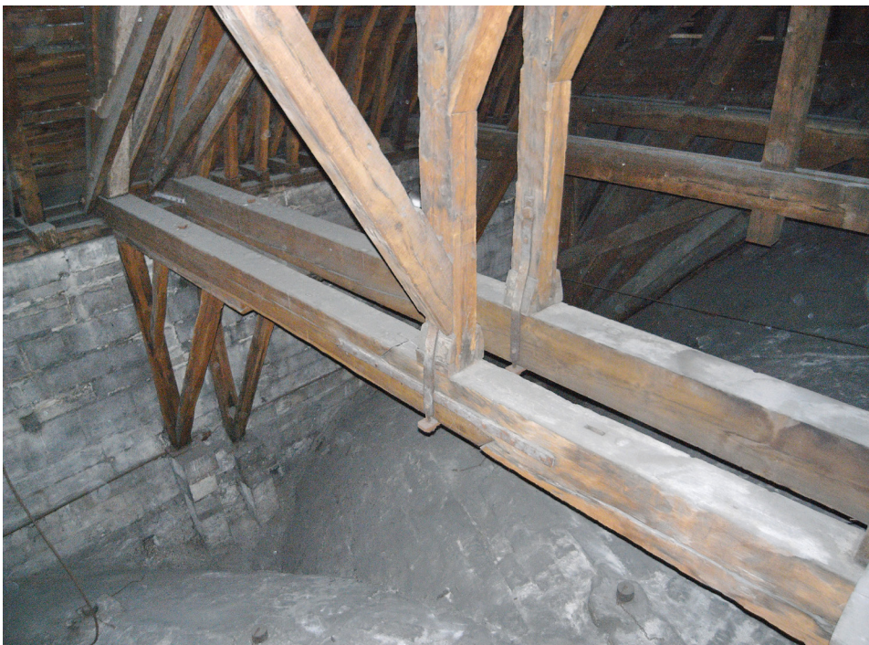
Fig. 2 A fragment of the Gothic structure of the roof truss of the Notre Dame cathedral in Paris, photo D. Mączyński 2009
