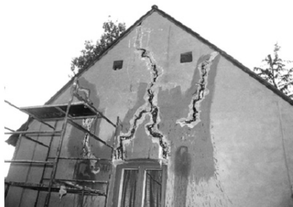
Figure 1. A detached house built in the area of intensive mining exploitation. Source: www.google.pl
