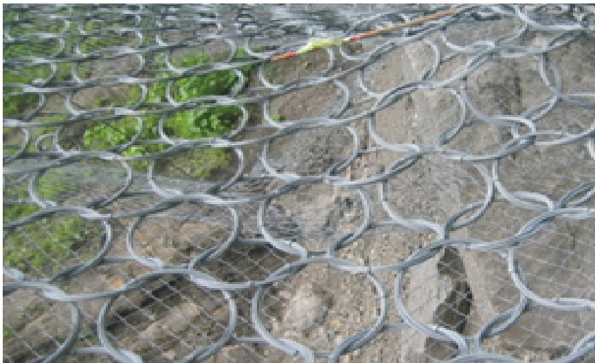
Figure 4. ROCCOR double steel net structure [6].
