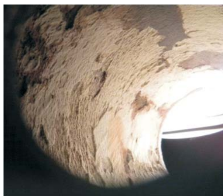
Figure 13. The interior of the position purified of the deposits after the application of EKOSTABIL. The picture was taken in the identical spot where the picture of Fig. 12.
