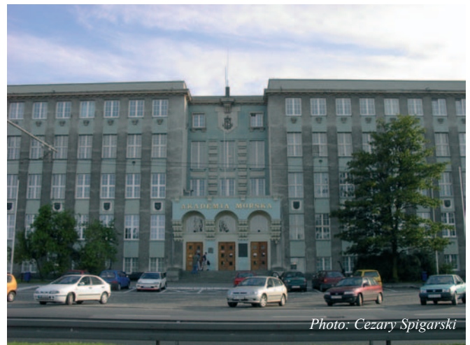
Main building of the Gdynia Maritime University .
