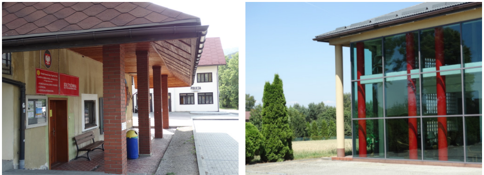
Fig. 11. Gutters obscuring turn points of roof (phot. M. Buško)
