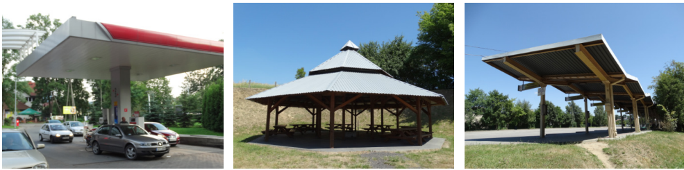
Fig. 12. Pavilions as specific types of buildings in Polish legislation (phot. M. Buśko)
