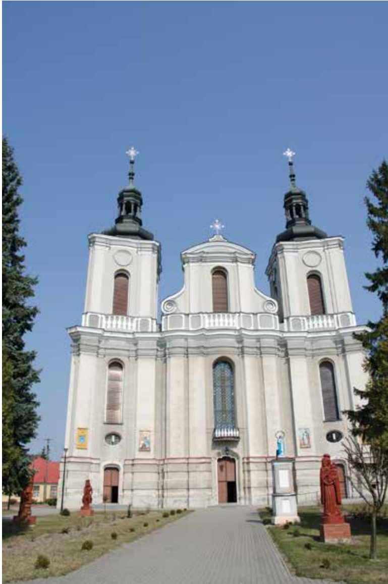
Fig. 13. The facade of the Calced Carmelite Church (2015), phot. Tomasz Rolski
