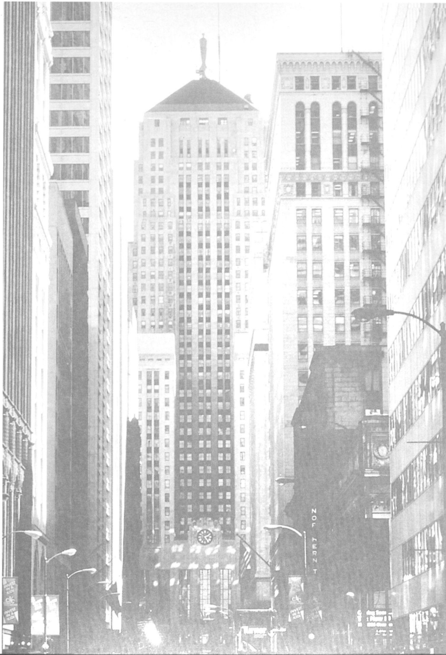
La Salle Street - Board of Trade Building
