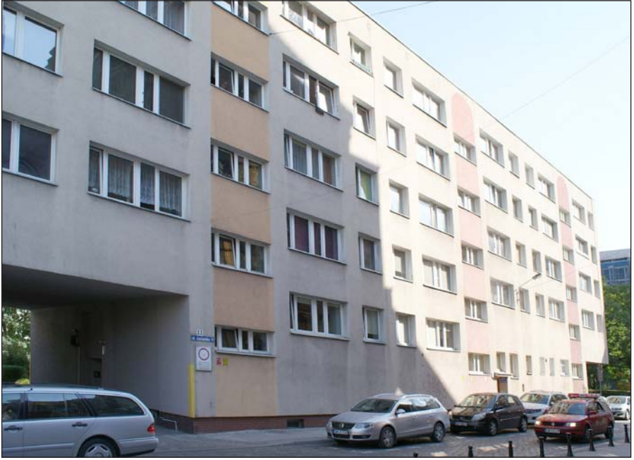
58. Façade from the side of 10-12 Łaciarska Street and a view from the kindergarten side (2018); photo: E.G.
