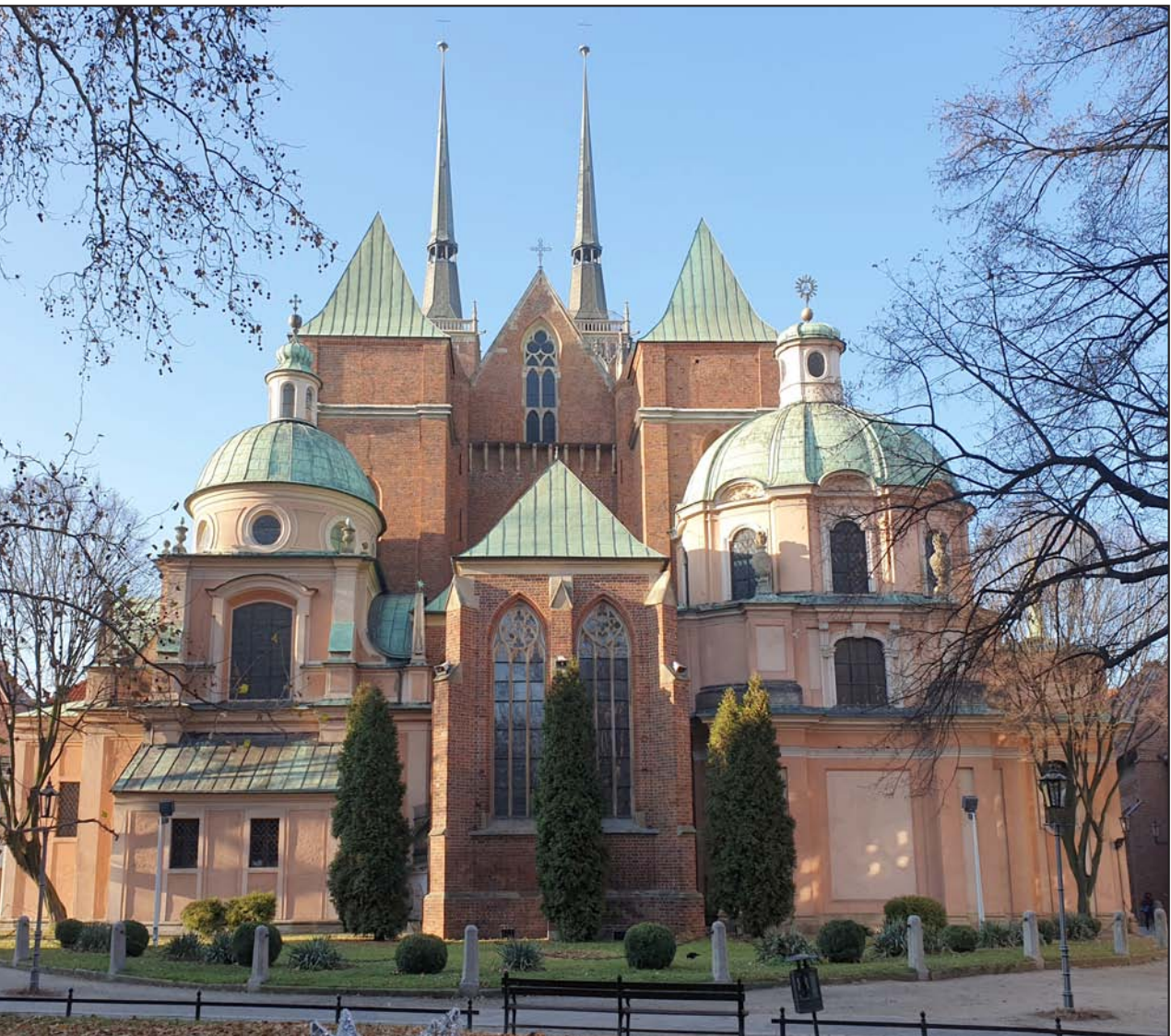
120. Eastern elevation of Wrocław Cathedral (2014); photo E.G.
