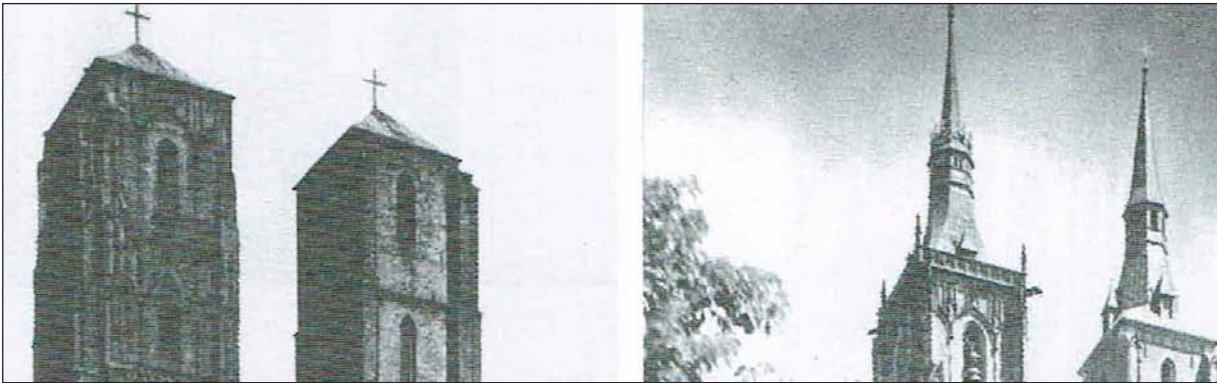
136. Tower spires of Wrocław Cathedral before and after restoration works were carried out (1908–1922) – so-called Hartung’s spires [79, p. 154]
