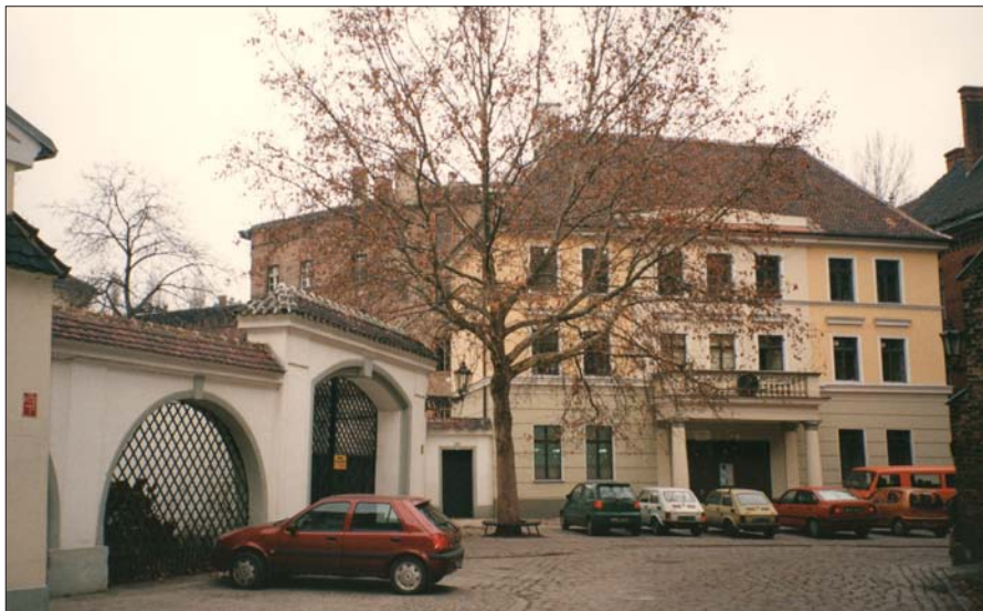
128. View of the southern elevation of the building at 11 Kanonia Street with a fence; from the archives of the Małachowicz family
